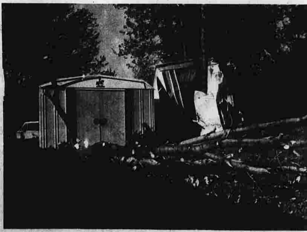
Crushed Shed on Phoenix St., Vernon
