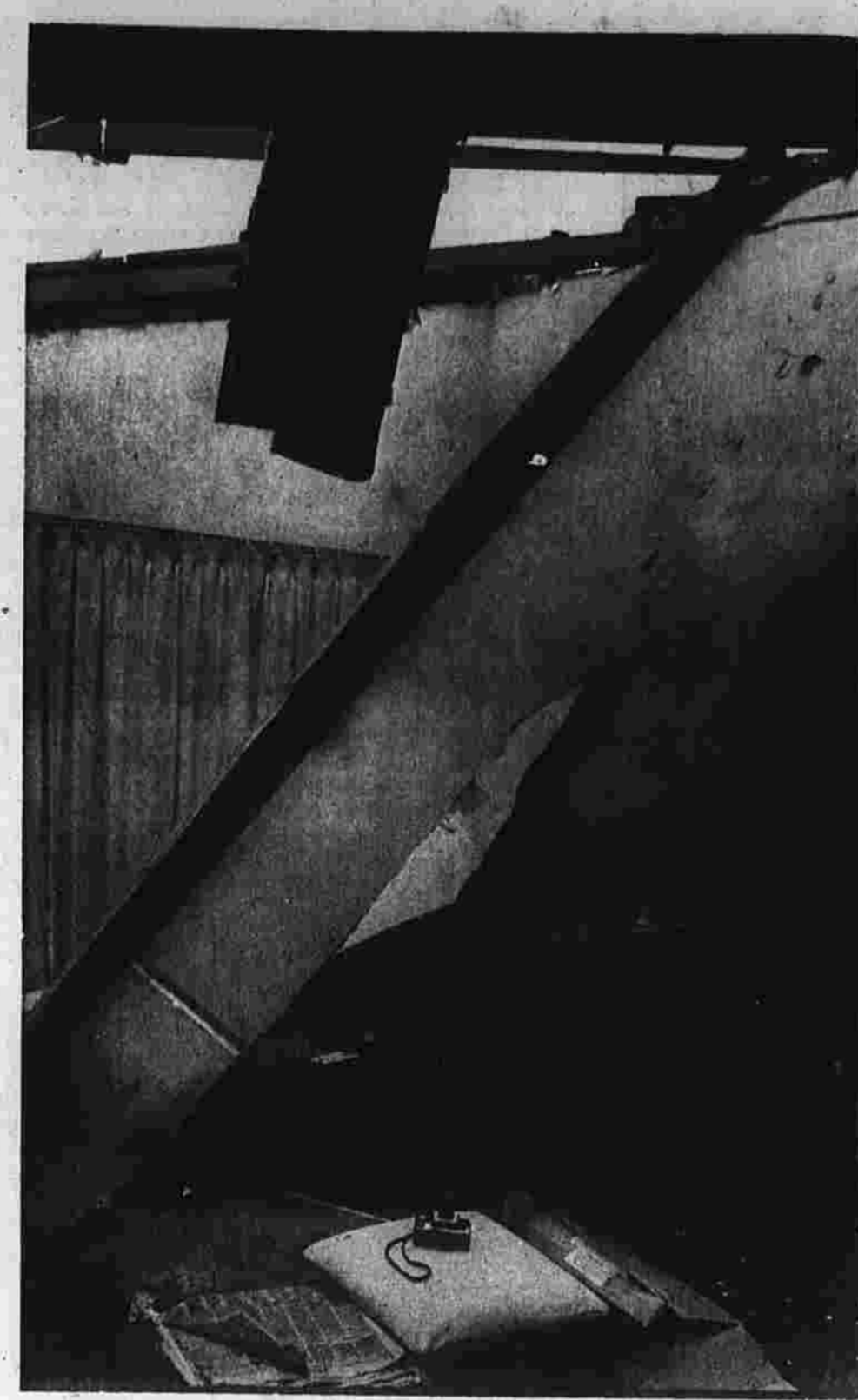
Inside Apartment at Oakland Manor
