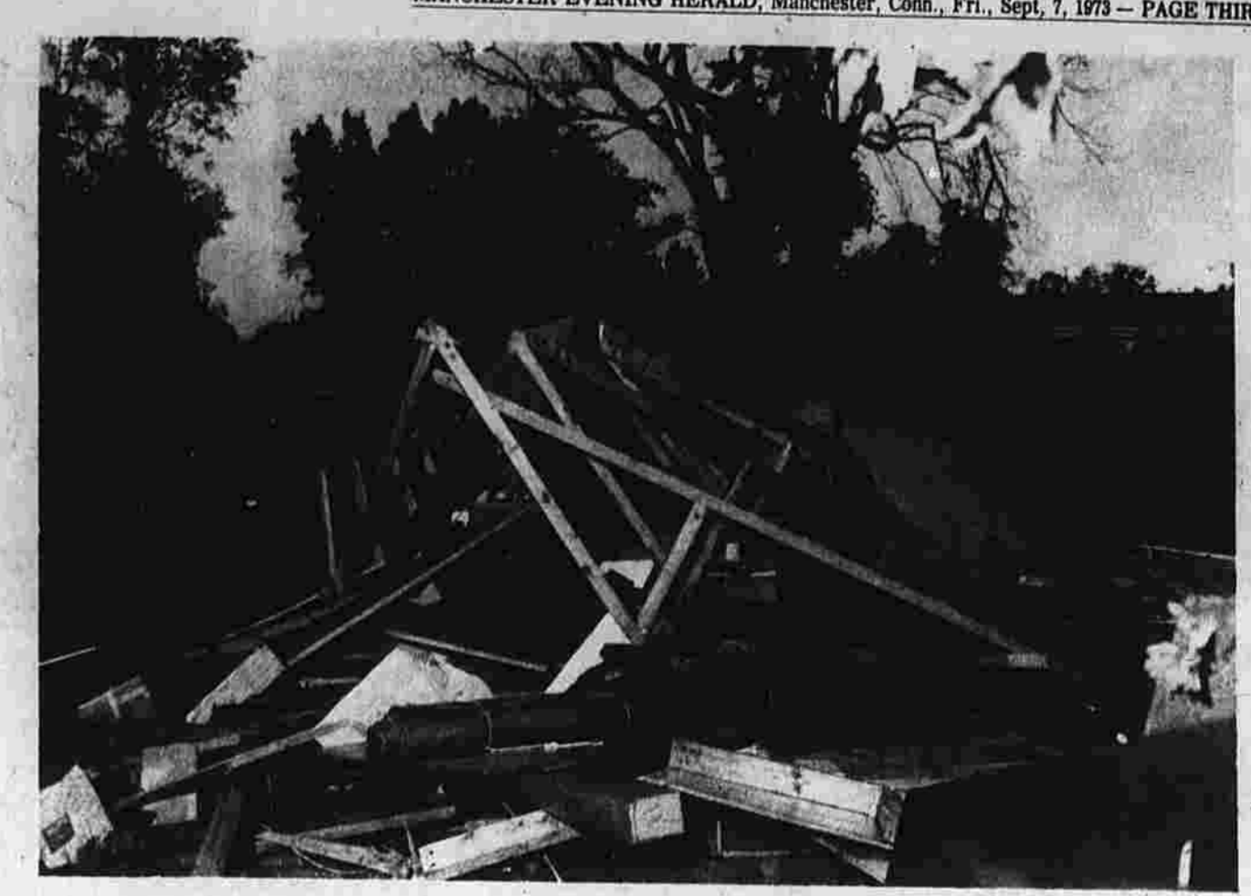
Roof of Garage at Oakland Manor Apartments
